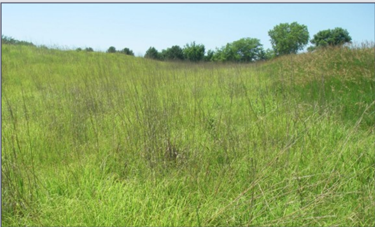
A well-maintained vegetated earthen spillway has a healthy, dense grass cover (no crops, vehicle ruts, or cattle paths) and smooth slopes (no abrupt transitions). Earthen spillways also must be kept free of obstructions that can collect debris and cause flow turbulence such as trees, fence lines, hay bales, and farm equipment.
