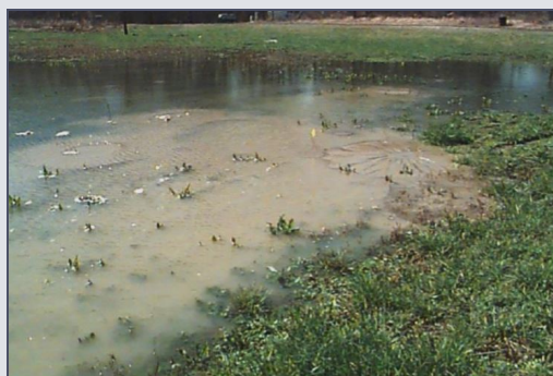
Severe example of a boil and seepage with significant cloudy flow. Cloudy flow is a sign that erosion is occurring inside a dam (Photo source: FEMA)
