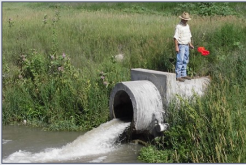
Spillway outlets must be free flowing to discharge water as designed.
