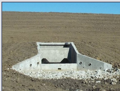
A well-designed plunge pool (left, right) or stilling basin (center) can prevent erosion at the outlet of spillway pipes.
