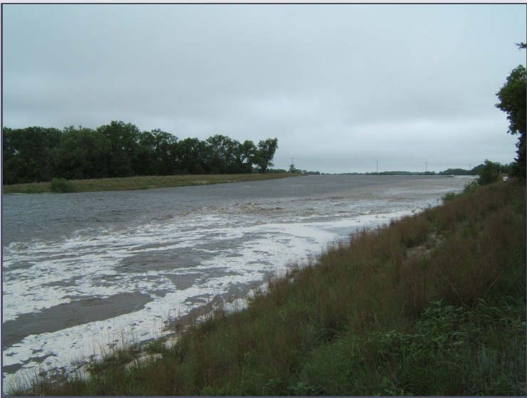
Auxiliary spillway flowing at a dam in Wheeler County. Spillways should be kept free of obstructions such as trees, posts, fence lines, and equipment that will catch debris and cause turbulent flow.
