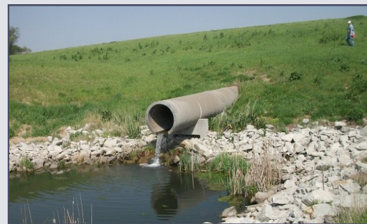
A well-designed plunge pool (left, right) or stilling basin (center) can prevent erosion at the outlet of spillway pipes.
