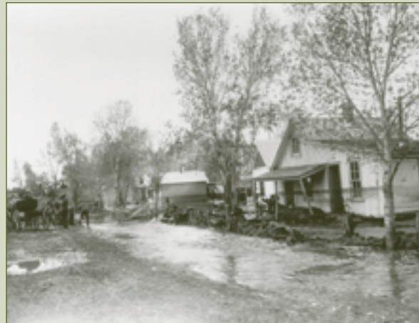
1904 flood damage in the Poudre River basin
