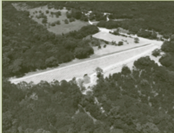
Oak Hill regional stormwater detention facility
