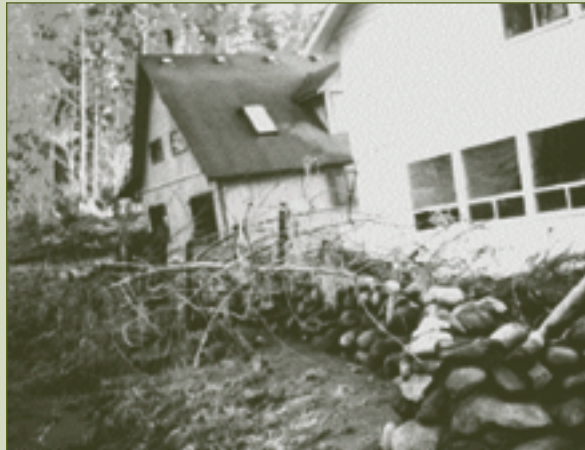
Nisqually Pines home pushed off its foundation
