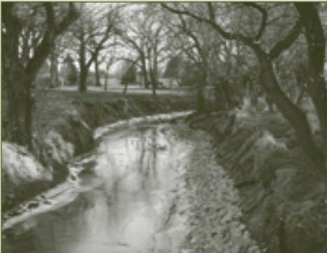
Streambank stabilization project
