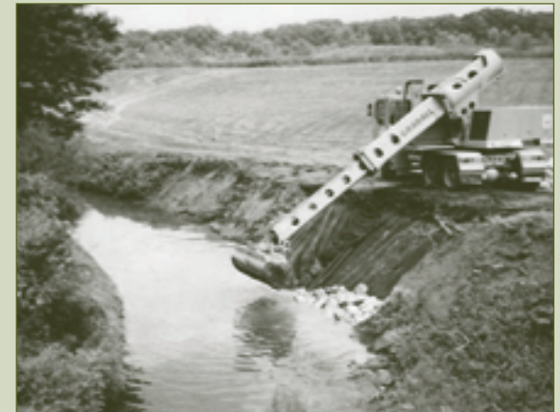
Thornton Ditch undergoing work
