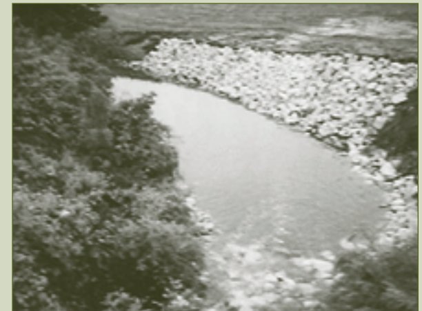
Thornton Ditch repaired
