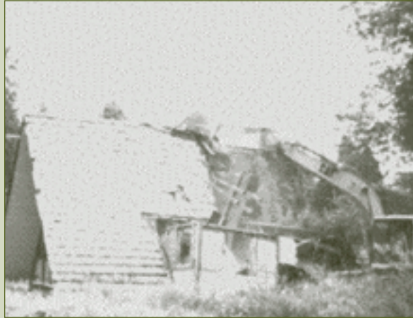
Demolition of damaged home at Hayco Lane
