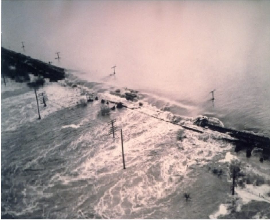
February 1986 Yuba River levee failure inundated the towns of Linda and Olivehurst, causing more than $400 million in damages. Image credit: David Rogers, University of Missouri-Rolla.
