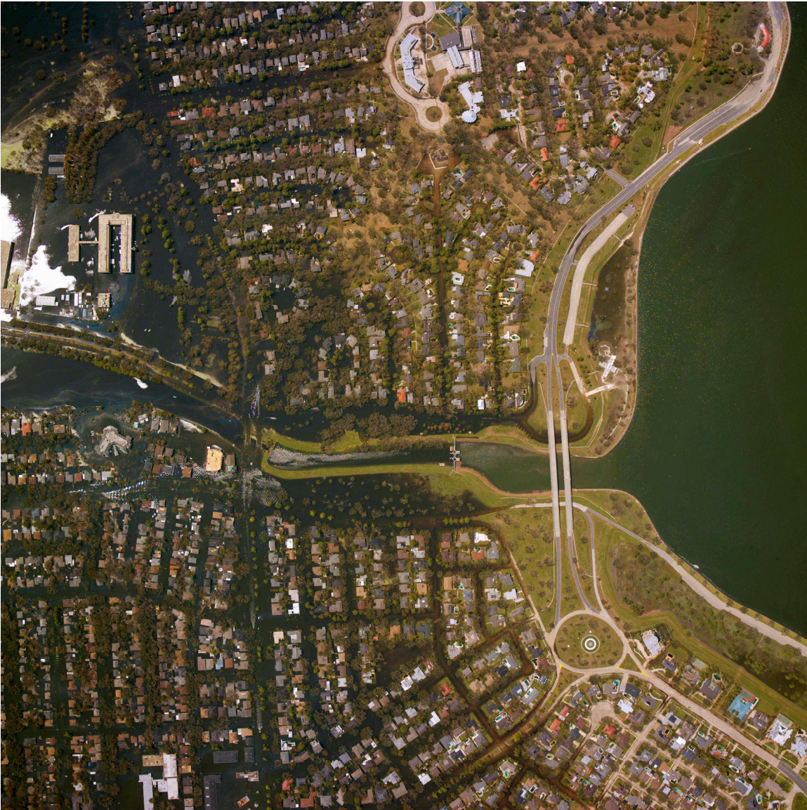
NOAA aerial survey of New Orleans on August 31, 2005, two days after Hurricane Katrina made landfall. Image credit: NOAA Navigational Response Teams.
