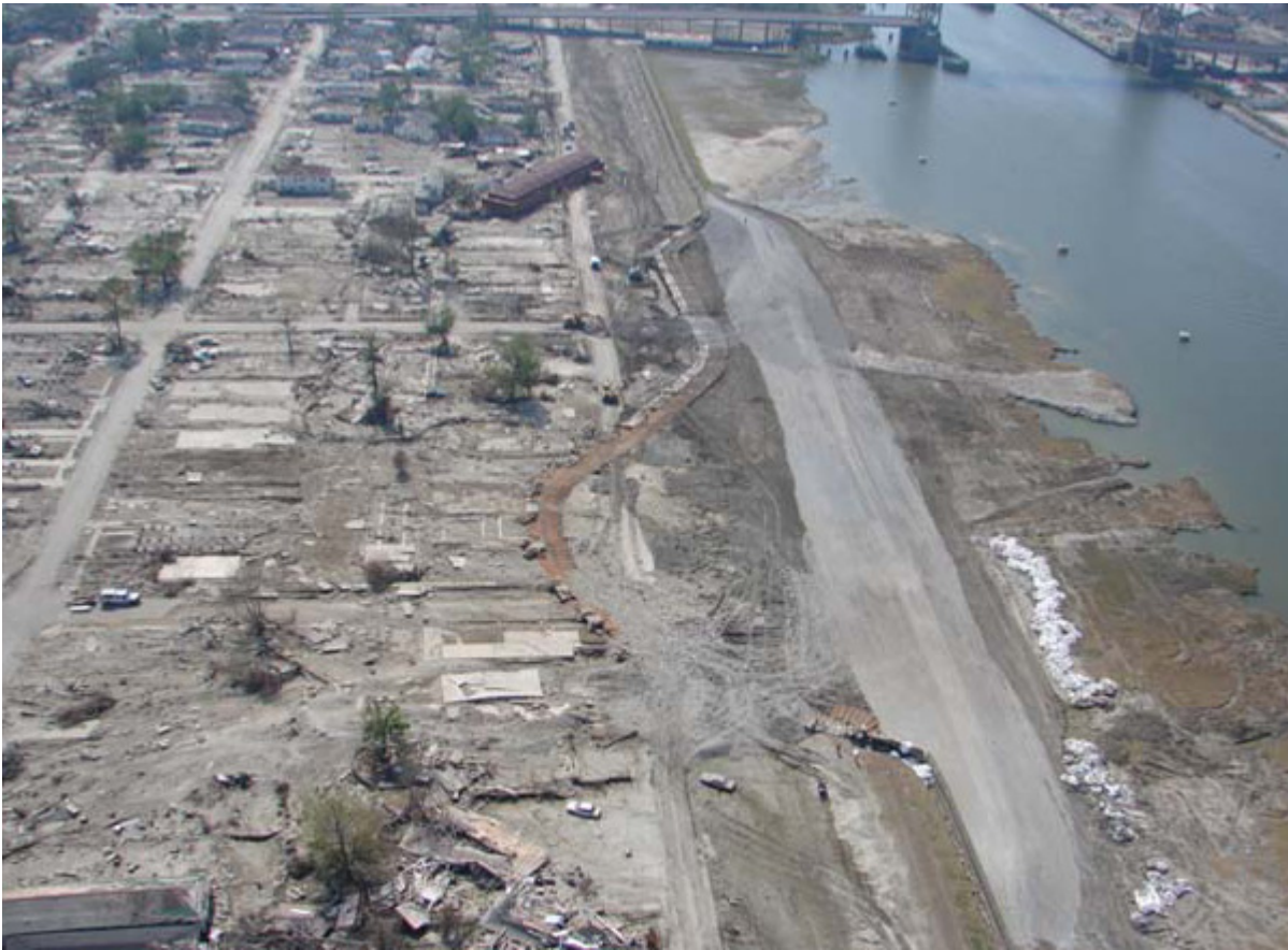
Oblique view of the (south) levee break at the Inner Harbor Navigation Canal into the lower Ninth Ward. Image credit: Leslie F. Harder for American Society of Civil Engineers.
