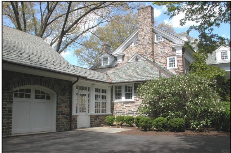
Photo 1. Example of Enclosed Breezeway.
