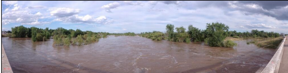
Figure 1. Before and during flooding view from bridge near Big Springs (NWS)
