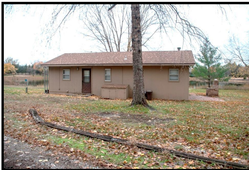
Figure 2. Homes like this one in Cedar Creek have their first floor 4 or 5 feet below the base flood elevation. Elevating this home would reduce flood risk, reduce flood insurance, and make the family safer.
