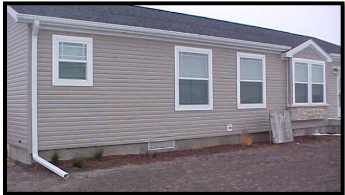
Figure 6. Flood vents on a rebuilt home in Pilger
