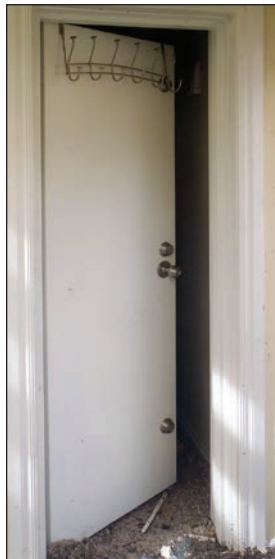
Residential safe room door (Moore, OK, 2013)
