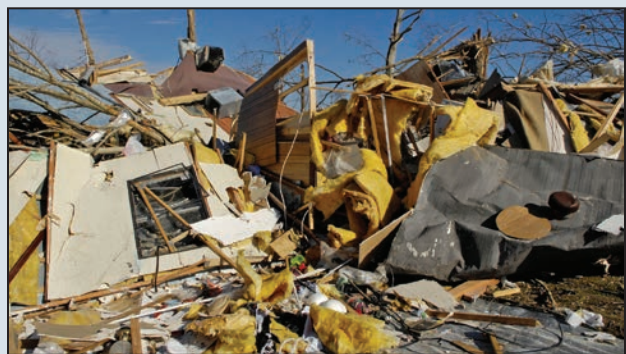
This photograph from FEMA's photo library shows the vivid reality of how lives are impacted by tornadoes (Lafayette, TN, February 5, 2008).
