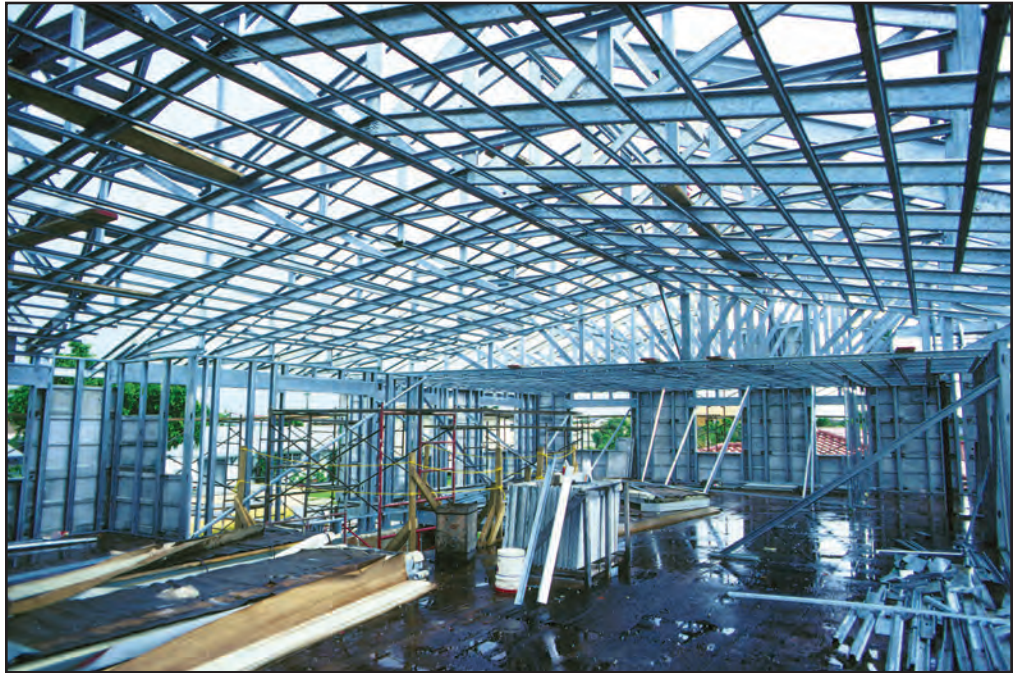
Figure 54 Metal framing is used for the new second story, including the walls and roof support system.
