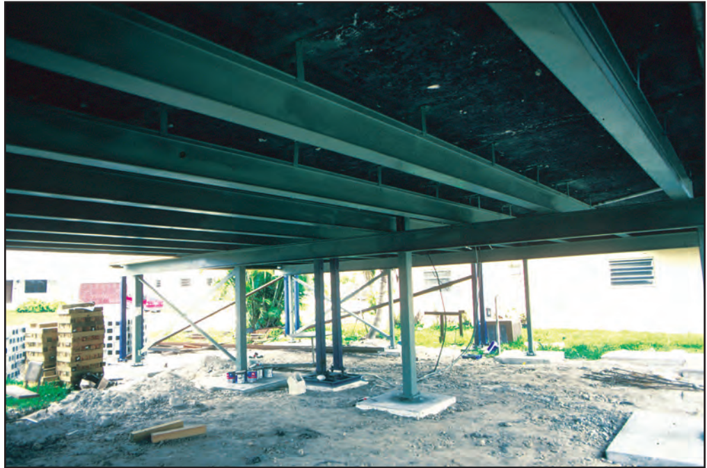
Figure 82 While the jacks and beams supported the house, new steel foundation members were installed below.
