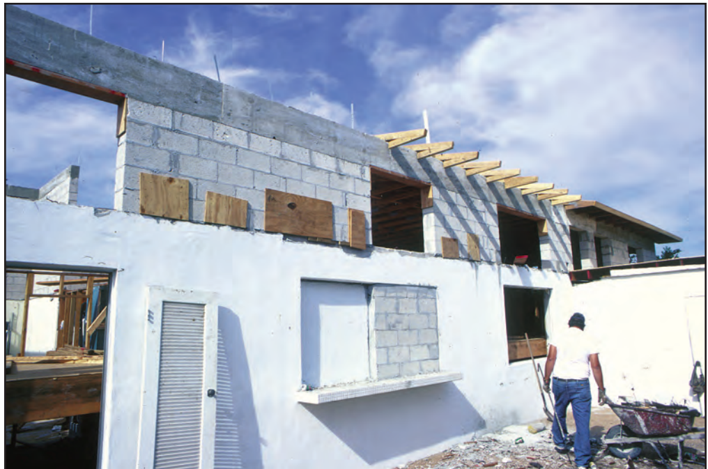
Figure 67 The extended first-story walls.
