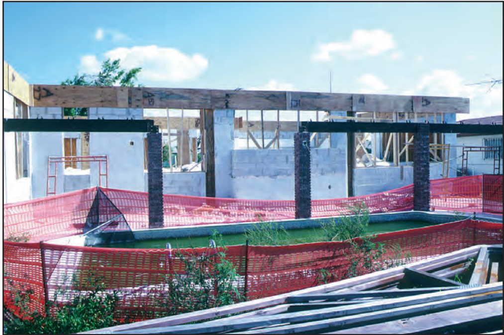
Figure 23 View from the back of the house. The walls have been extended upward with concrete blocks. The plywood visible at the tops of the walls is used to form cast-in-place concrete bond beams that will strengthen the extended walls. The roof trusses shown in the foreground were salvaged for reinstallation. The owner of this house decided to replace the original roof sheathing and shingles with new materials.
