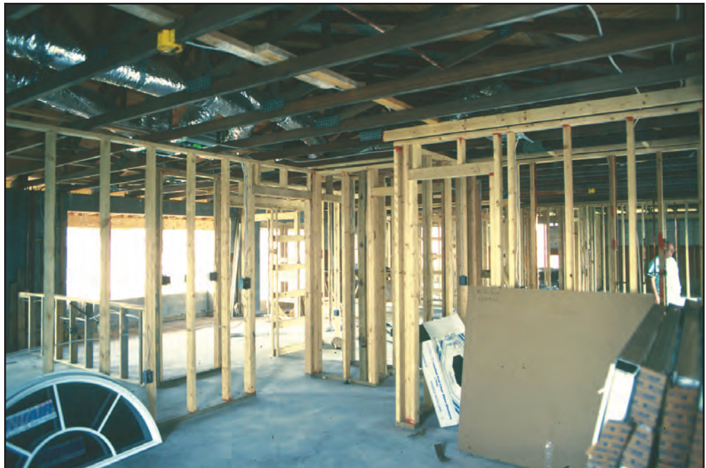
Figure 30 Interior partition walls and utilities are added.
