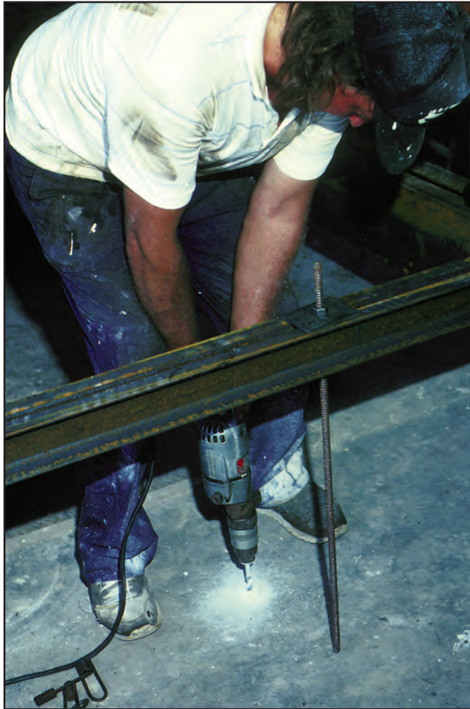
Figure 77 ... install anchors ...
