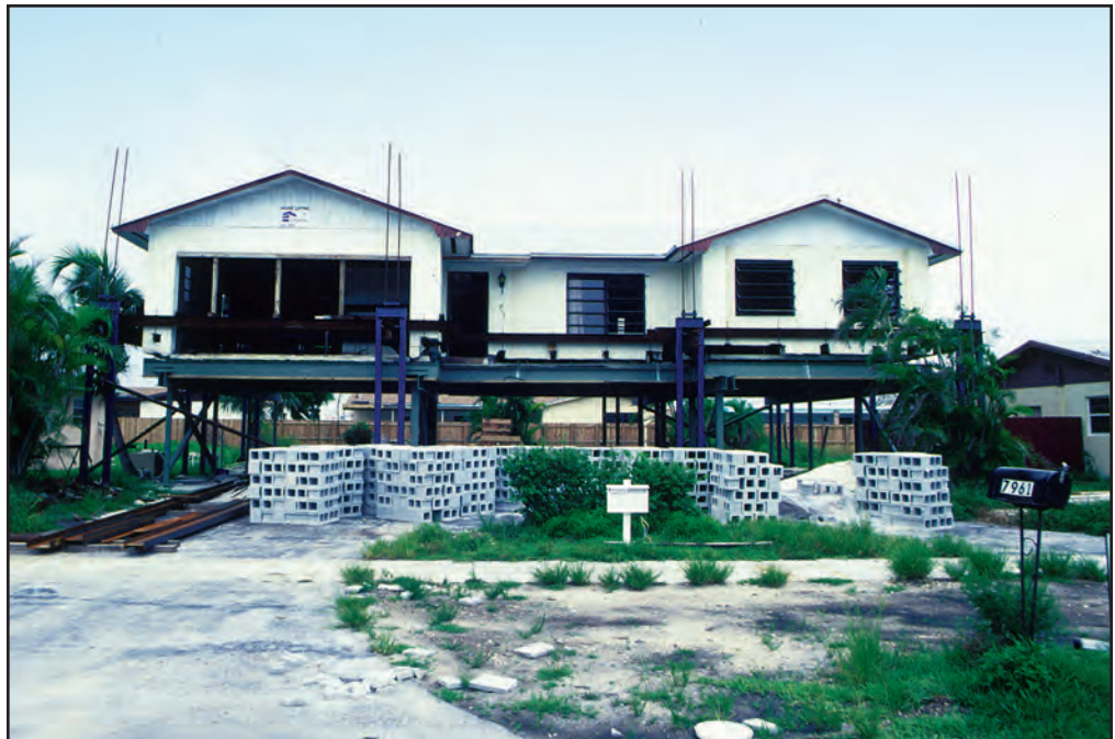
Figure 83 Concrete blocks were brought to the site ...
