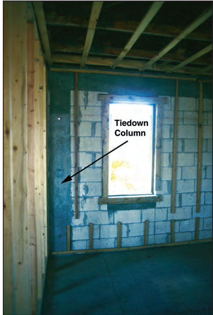
Figure 46 Concrete tiedown columns, such as the one to the left of the window in this photograph, were also used in this house.
