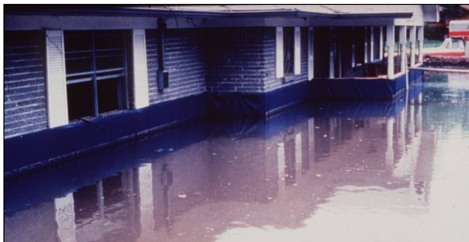
Figure 7-2. Photograph of membrane providing flood protection
