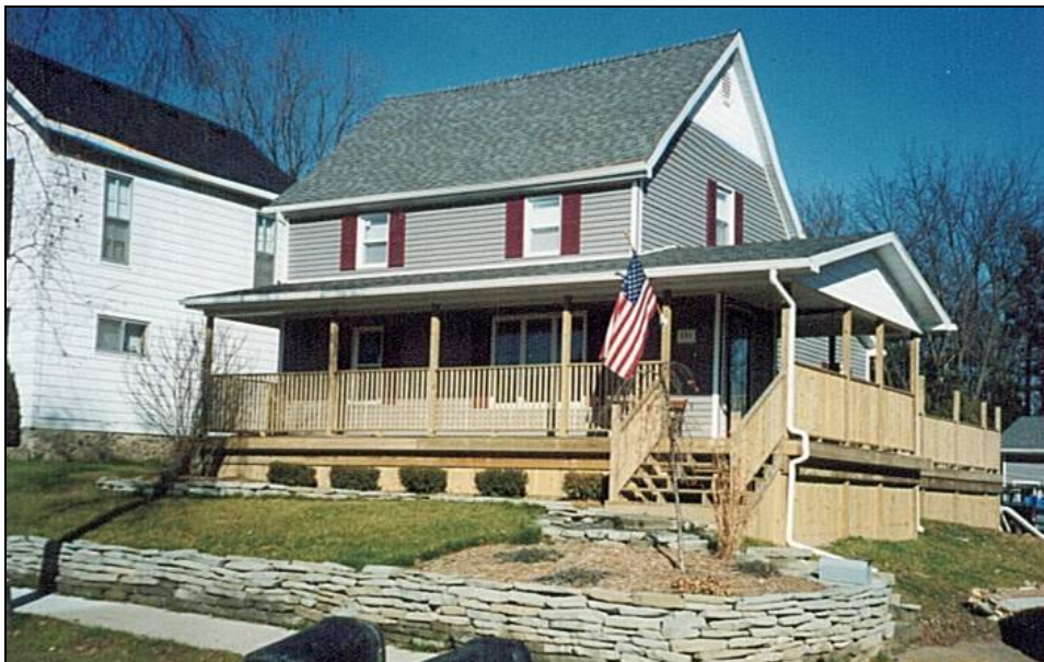
Figure 8-2. Residence shown in Figure 8-1 now elevated 5 feet
