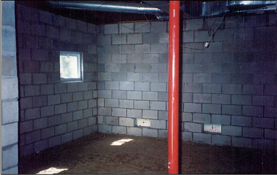
Figure 8-4. New foundation with vents
