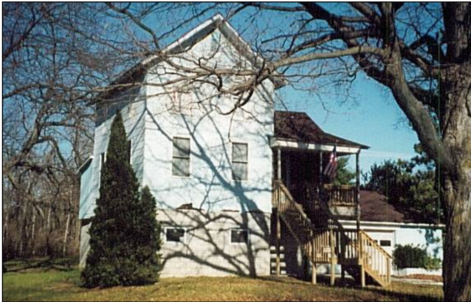
Figure 8-8. House elevated 8 feet, but lacking landscaping, producing a stark look
