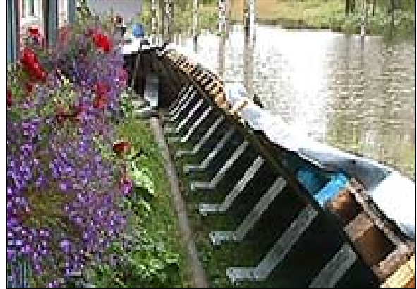
Figure 5-5. Metal supports for floodwall installed for deployment. Floodwall deployed with impermeable membrane.
