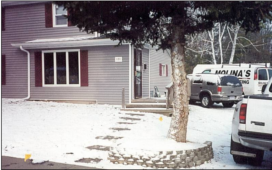
Figure 8-1. Residence before elevation
