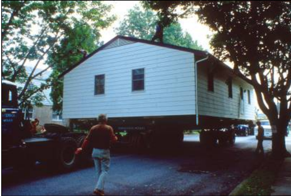
Figure 9-1. Structure placed on a wheeled vehicle for relocation to a new site
