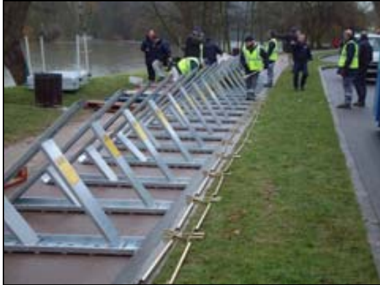
Figure 5-5. Metal supports for floodwall installed for deployment. Floodwall deployed with impermeable membrane.
