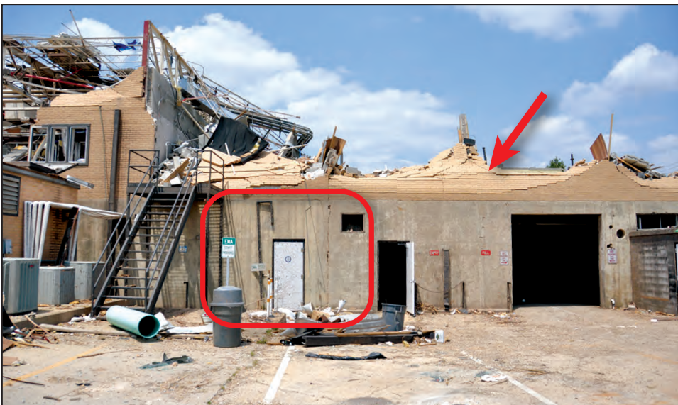
Figure B3-14. Collapse hazard: the story above an Emergency Operations Center collapsed. Masonry walls (red arrow) and part of the roof structure fell onto the second story floor slab above the EOC (Tuscaloosa, AL, 2011 tornado)
