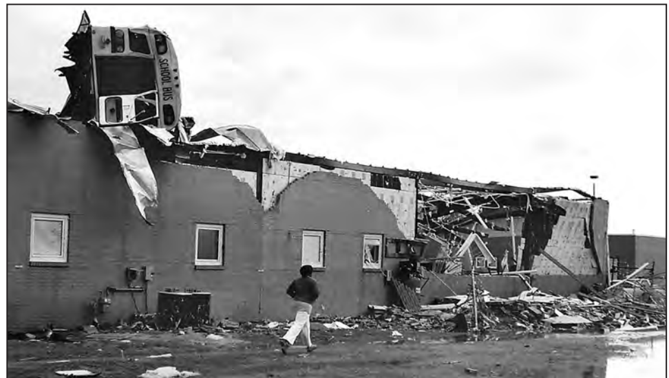
Figure B8-8. Large debris: A school bus was lifted atop a school. (Caledonia, MS, tornado, 2008)
