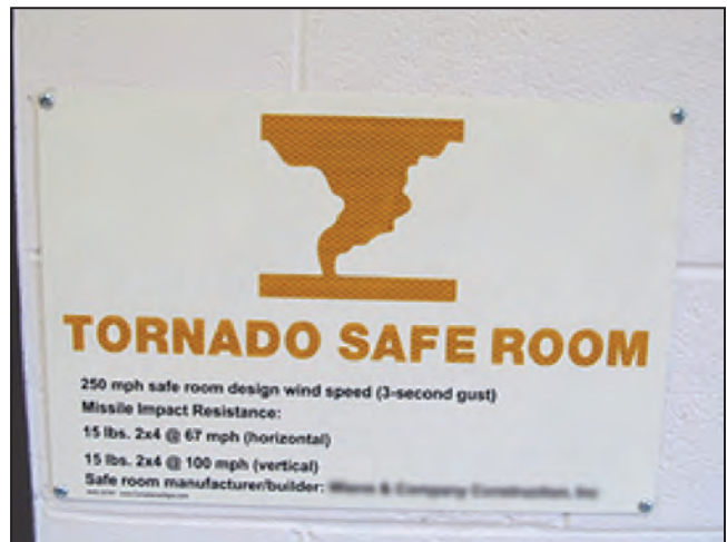
Figure B1-6. Examples of design information signs; though these include Missile Impact Resistance information, such information is not required
