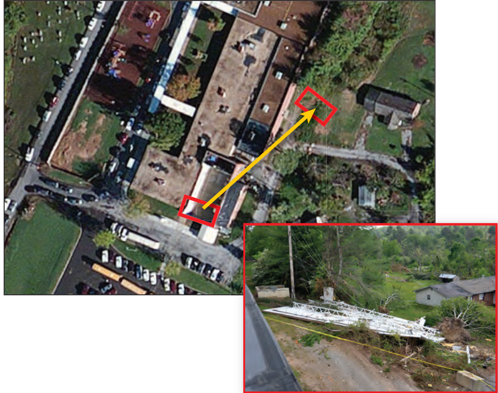
Figure B3-15. Flying debris hazard: an EF1 tornado blew a school gymnasium's steel truss and steel deck roof assembly approximately 230 feet (Cleveland, TN, 2011)
