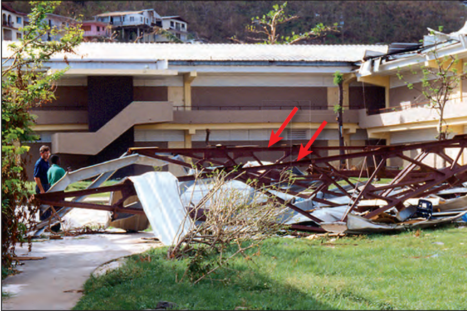
Figure B8-5. Large debris: Steel roof trusses that blew off a school (U.S. Virgin Islands, 1995 Hurricane Marilyn)
