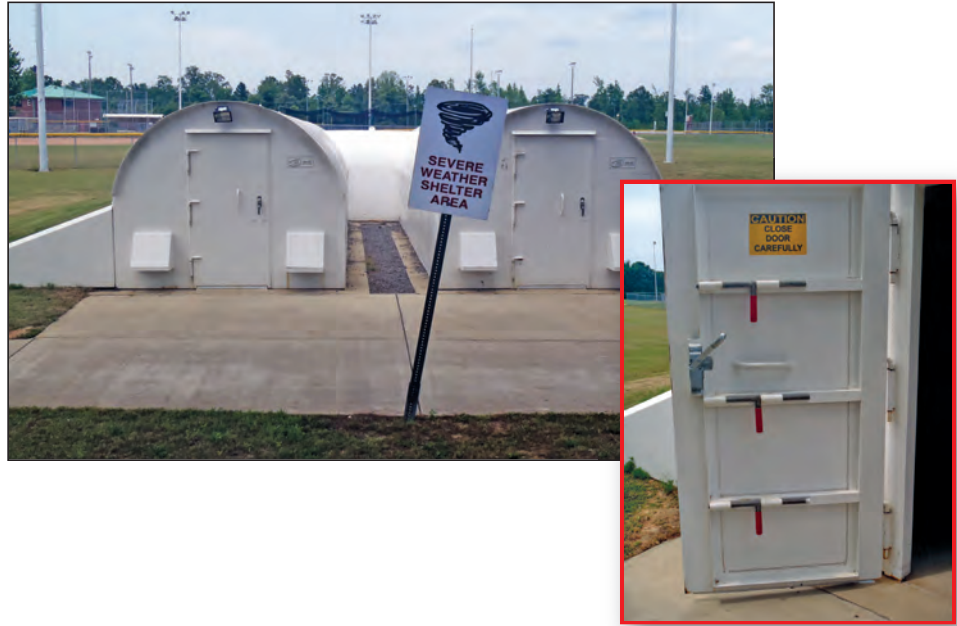
Figure B1-2. Prefabricated steel single-use community safe room (Brookwood, AL)
