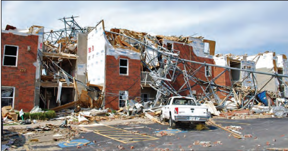
Figure B3-12. Lay down hazard: failure of a large communications tower onto a building (Joplin, MO, 2011 tornado)
