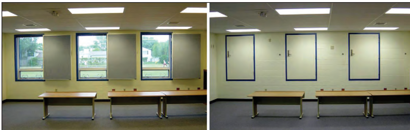
Figure A4-5. Interior operated safe room shutters in multi-purpose classroom/safe room. Image on left is normal usage; image on right shows shutters in 'lock down' position where they are closed and latched
