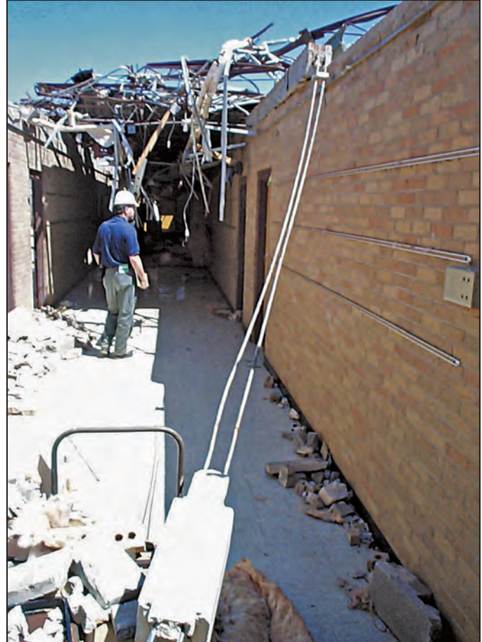
Figure B3-8. Load path failed between the bond beam and the top of the unreinforced masonry wall when struck by an F4 tornado (Moore, OK 1999)
