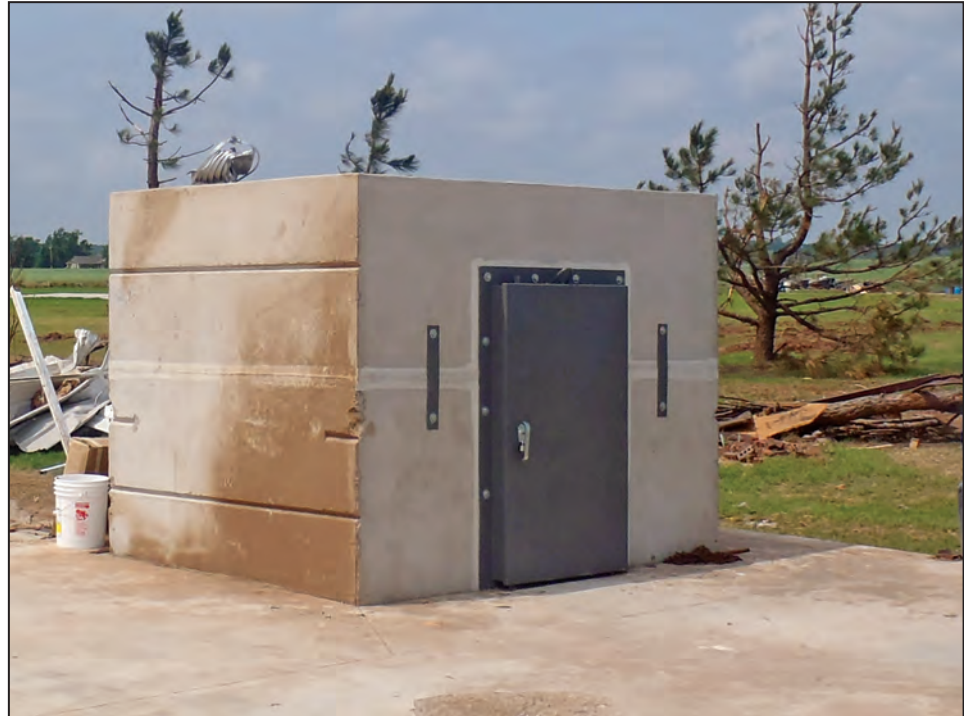
Figure B1-3. Single-use residential safe room after an EF5 tornado (Newcastle, OK)
