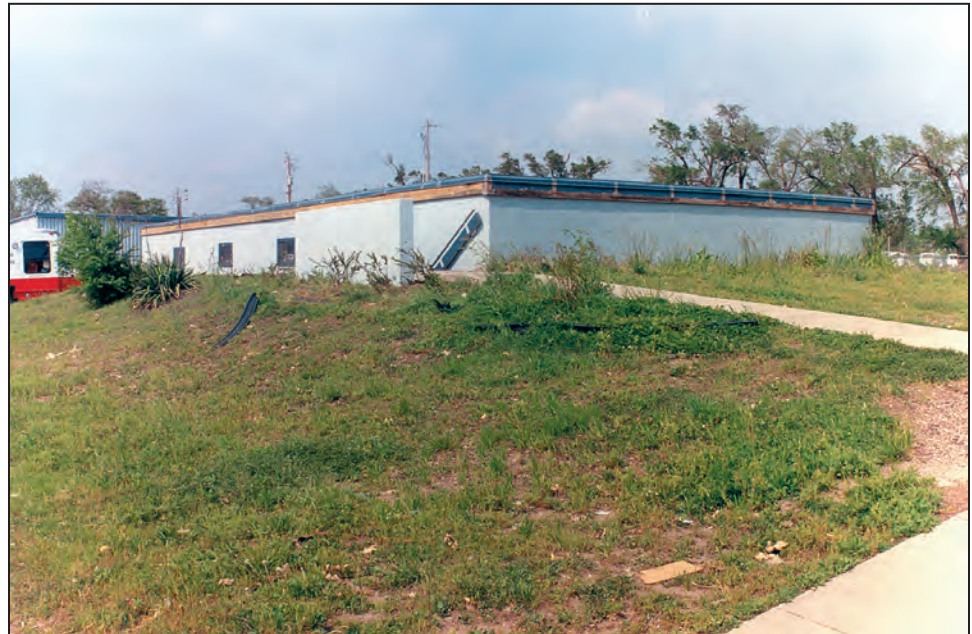
Figure B3-10. View of a community shelter that is partially below grade (Wichita, KS, 1999 tornado) (SOURCE: FEMA P-342)
