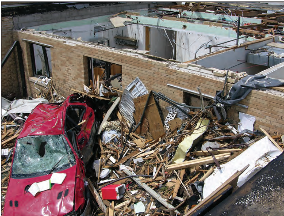
Figure B8-10. Representative quantity, size, and type of debris that is often generated by a strong or violent tornado. The building damage at this site was indicative of an EF3 tornado. (Greensburg, KS, 2007)
