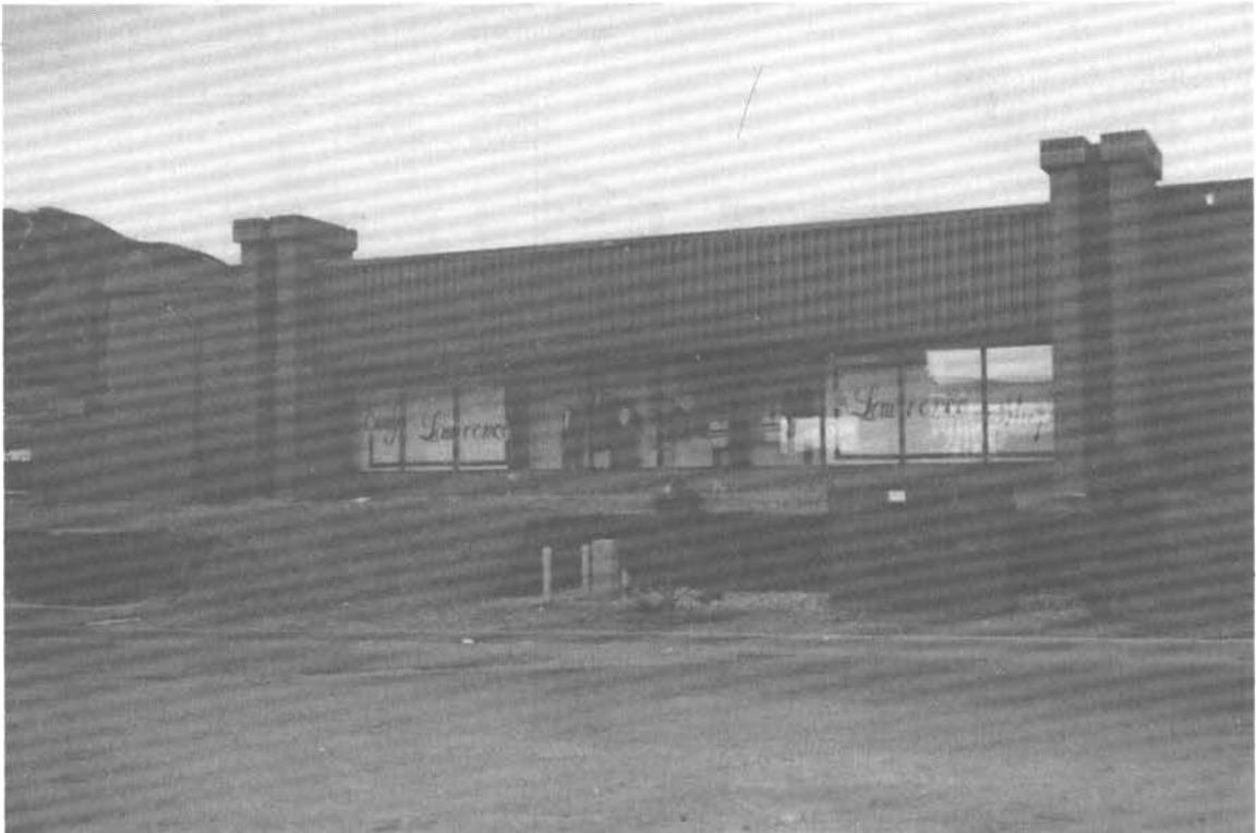
Figure I-8. Elevation on Compacted Fill
