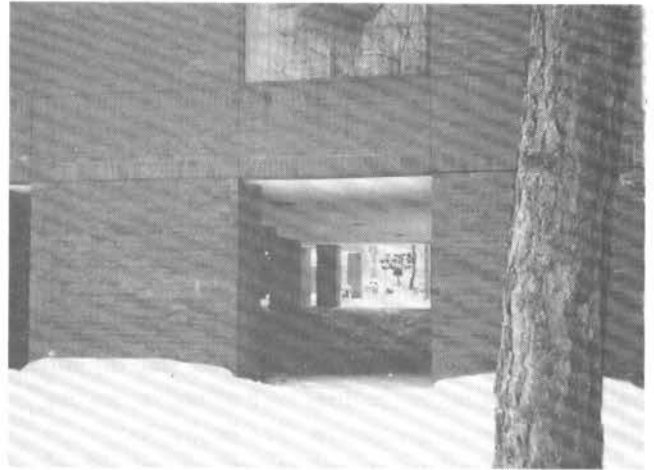
Combined use of wall and columns minimize visual impacts of 12 foot elevation height.
