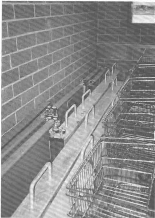
Stored flood shields (Note pneumatic seal valves).
