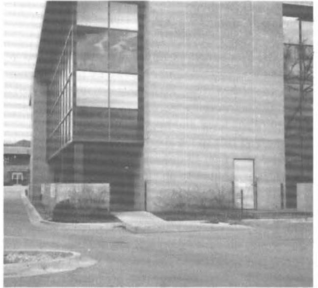
Structure can be floodproofed with a total of 5 flood shields.
