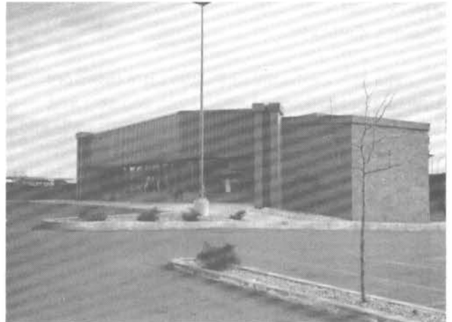
Site grading provides direct access to first floor elevation at the front of the structure.
