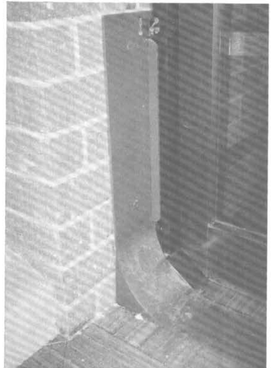
Detail of frame used for mounting shield at front door.
