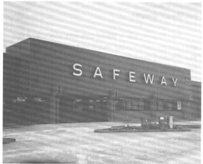
Existing Safeway Building has been retrofitted with flood shields to protect against flood depths up to 2 feet above the 1st floor elevation.
