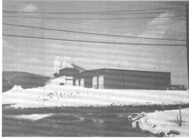
Garage structure elevated on earth fill.
