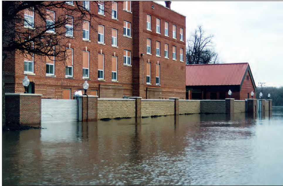
Figure 4-1. Typical masonry floodwall with engineered closures, which protected the Oak Grove Lutheran School in Fargo, ND, from flooding in 2001 (source: Flood Control America, LLC)
