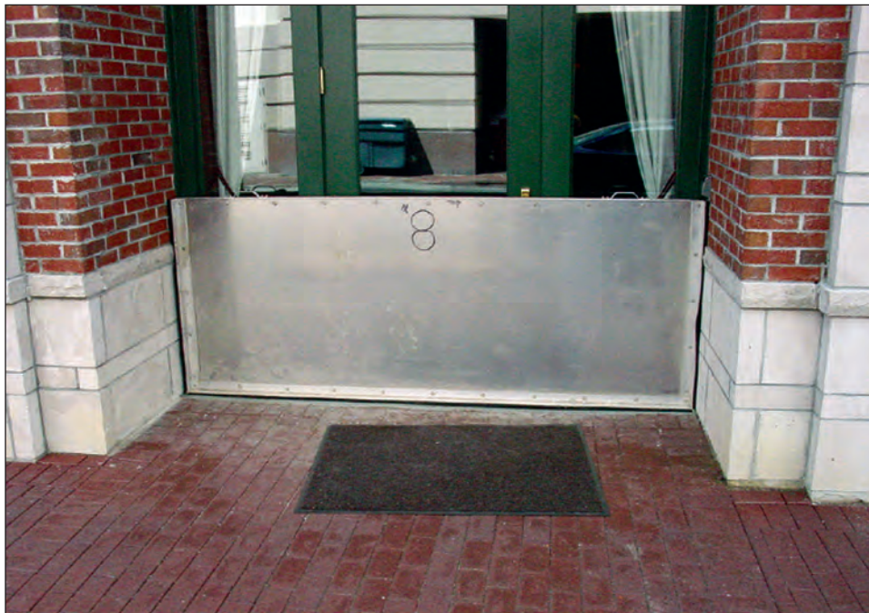
Figure 3-9. Aluminum flood shield used for flooding less than 3 feet deep
