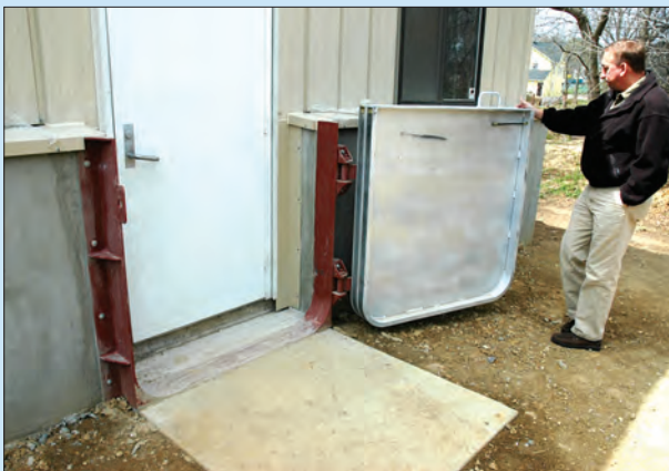
Figure 3-13. Rear of retrofit dry floodproofed building with permanently installed flood shield
