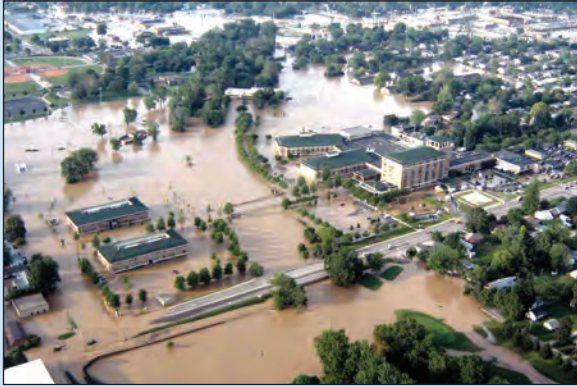
Figure 4-7. Floodwaters surround Columbus Regional Hospital in 2008
