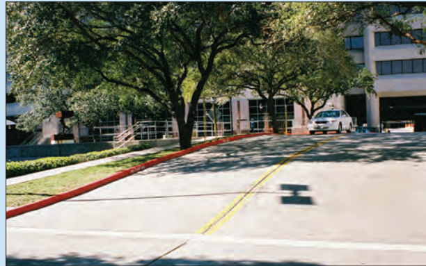
Figure 3-24. Ross Sterling Avenue was raised to protect the MSB to the level of the base flood (source: Walter P. Moore)
