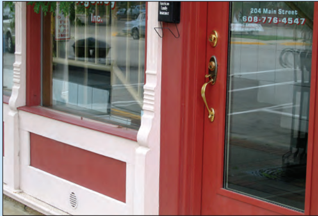
Figure 4-31. Businesses along Main Street in Darlington, WI, mitigated with an elevated interior first floor
