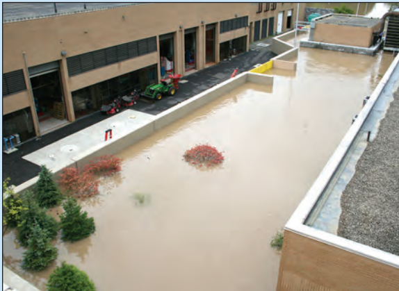
Figure 4-5. Floodwall successfully safeguards Lourdes Hospital from Tropical Storm Lee flooding (source: FloodBreak)
