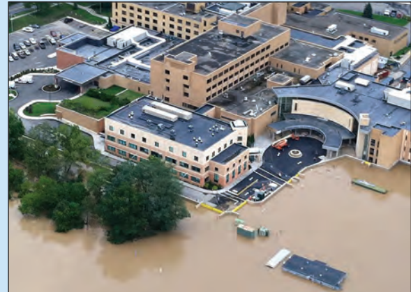
Figure 4-6 Aerial view showing effective protection of Lourdes Hospital from flooding as a result of Tropical Storm Lee
