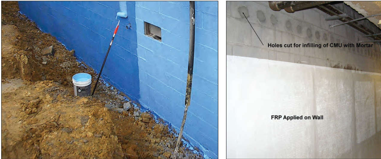
Figure 3-2. Application of a waterproof membrane on the exterior (positive side) of a wall (left) and fiber-reinforced polymer wrap applied to the interior (negative side) of a wall (right)
