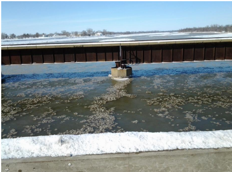
Sarpy County: Platte River Bridge Hwy 6
