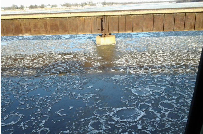
Sarpy County: Platte River Bridge Hwy 6
