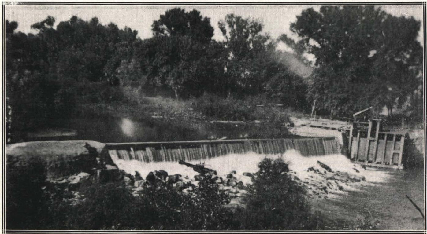
Power Development on Little Blue River at Fairbury
