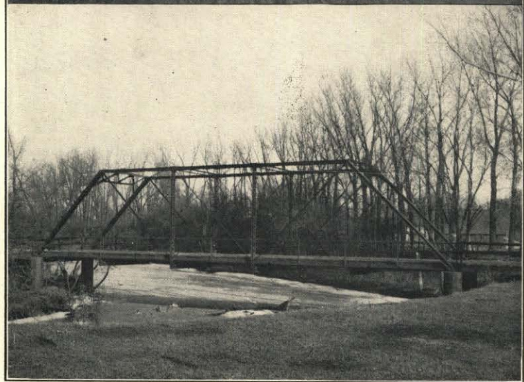
HIGHWAY BRIDGE, MADISON COUNTY. STATE ENGINEER'S OFFICE, 1906.
