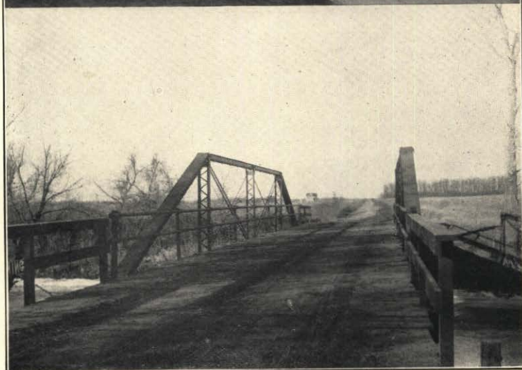
HIGHWAY BRIDGE MADISON COUNTY. STATE ENGINEER'S OFFICE, 1906.
