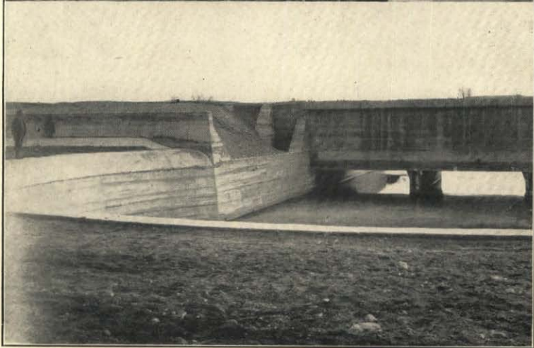
FLUME ON INTERSTATE CANAL.
