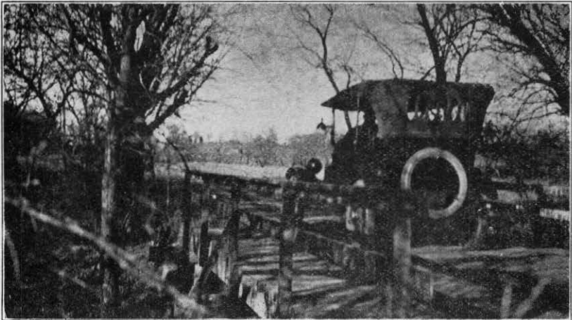
Old Type of Wooden Bridge Being Replaced by Permanent Structure.
