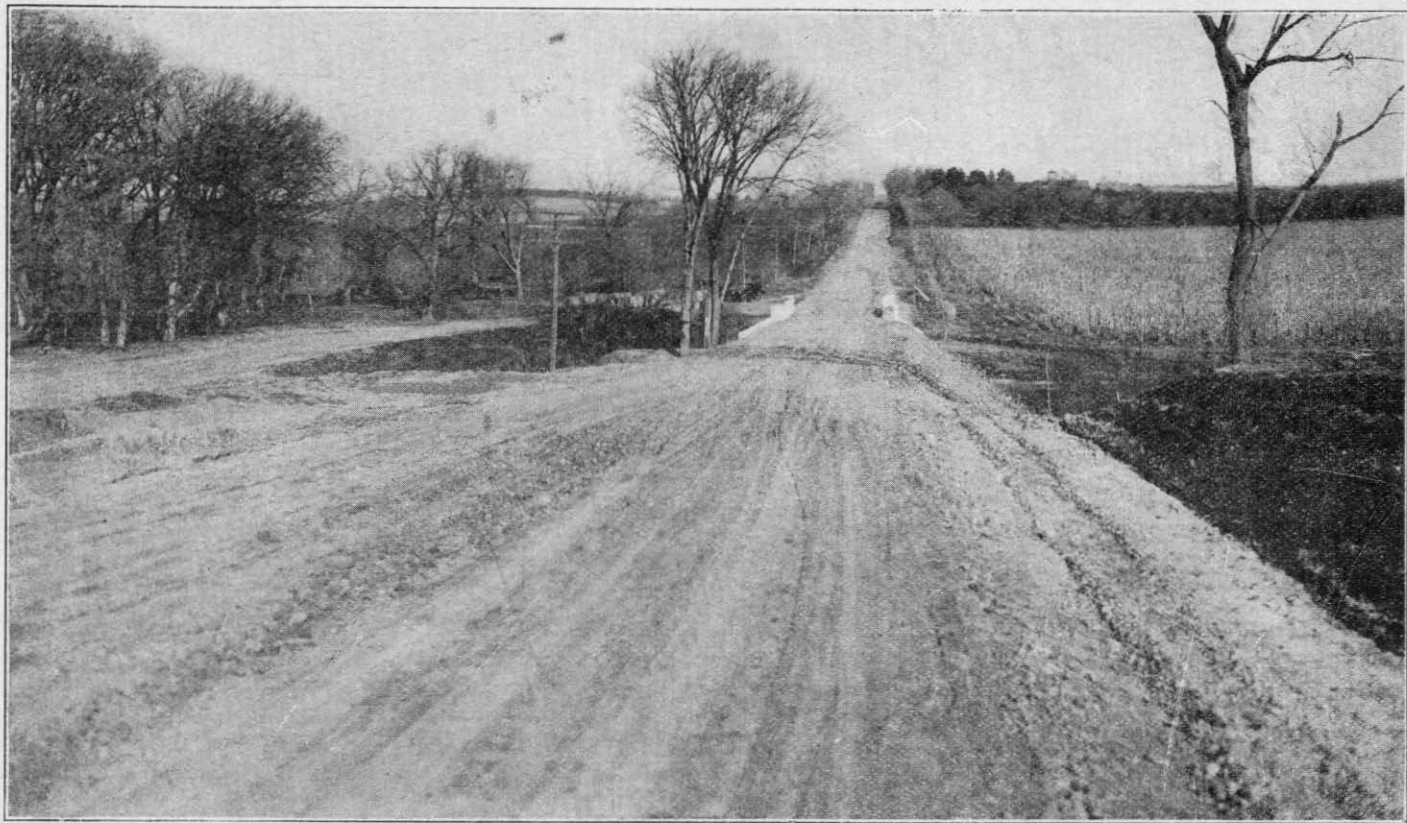
Elimination of a Dangerous Curve in Otoe County. Federal and State Aid Project No. 7.
