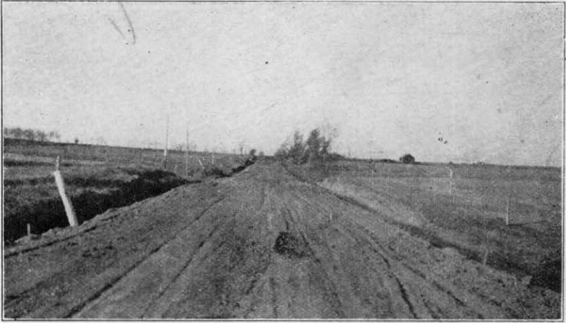
Ufinished Road, Adams County Work Only Started on this—Project No. 7
