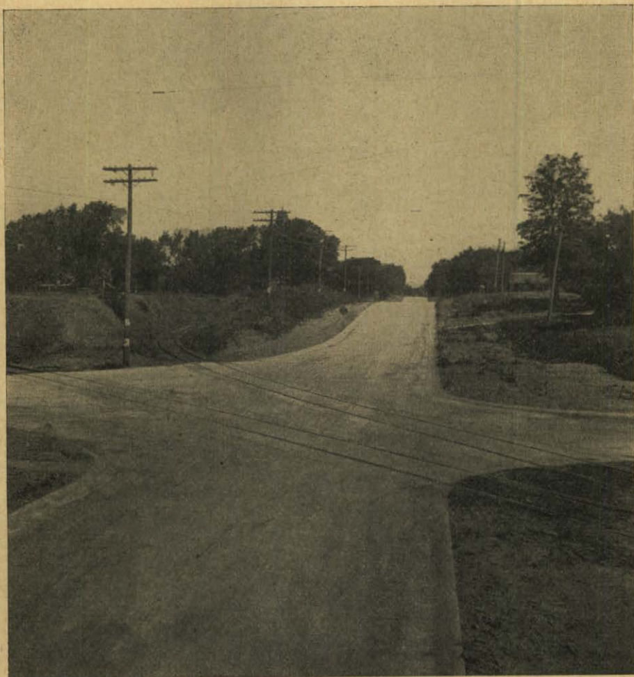
The above view shows a concrete pavement through the west part of Wahoo, Saunders County, missing the main business street and saving two right angle turns. Built with Federal, City and State Funds in 1927.
