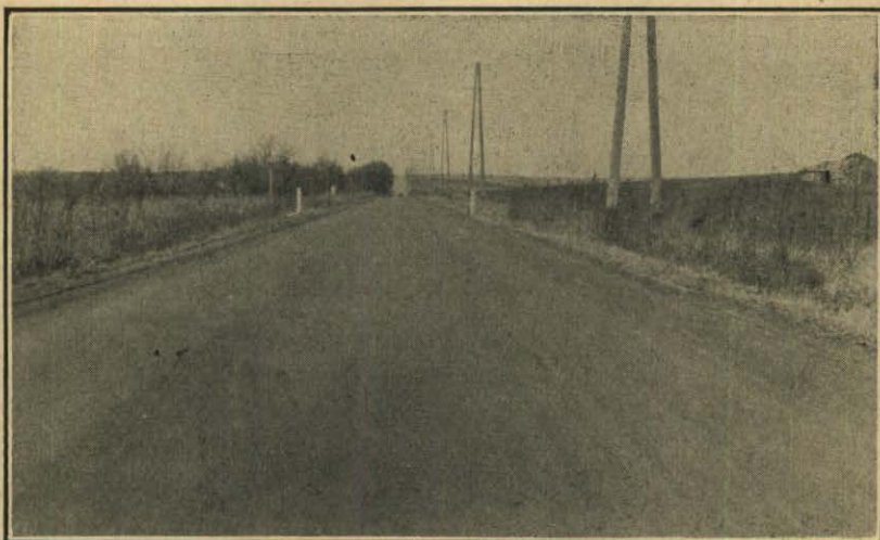
Oiled gravel on the Cornhusker Highway seven miles north of Lincoln, Lancaster County.
