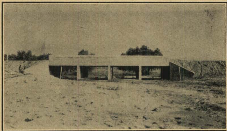
Quadruple 12x8x32 Foot Concrete Culvert. Project No. 205-D.
