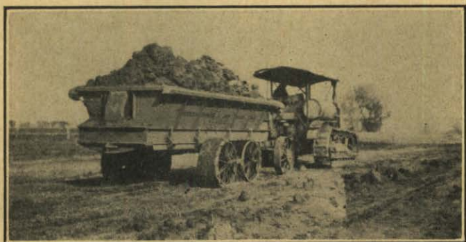
Hauling embankment material on the Ames-North Bend project, Dodge County.
