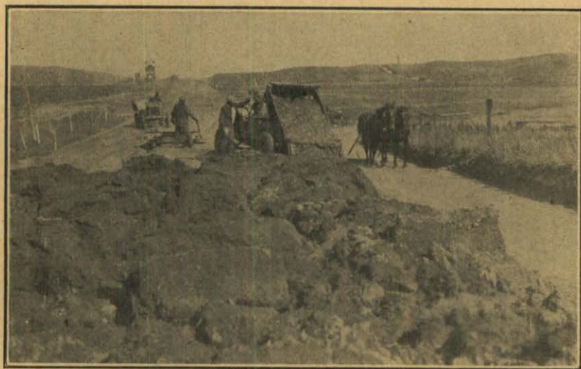
Drag-line work thru lake in Lakeside-Ellsworth project. This is the kind of material also used to cover the sand base as shown in the picture below.
