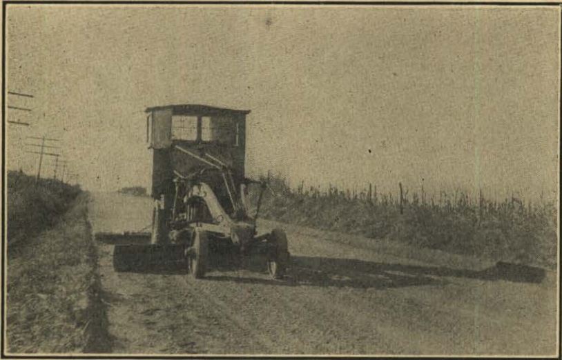
A "One Man" blade unit pulling drag behind, gives double maintenance with one trip.
