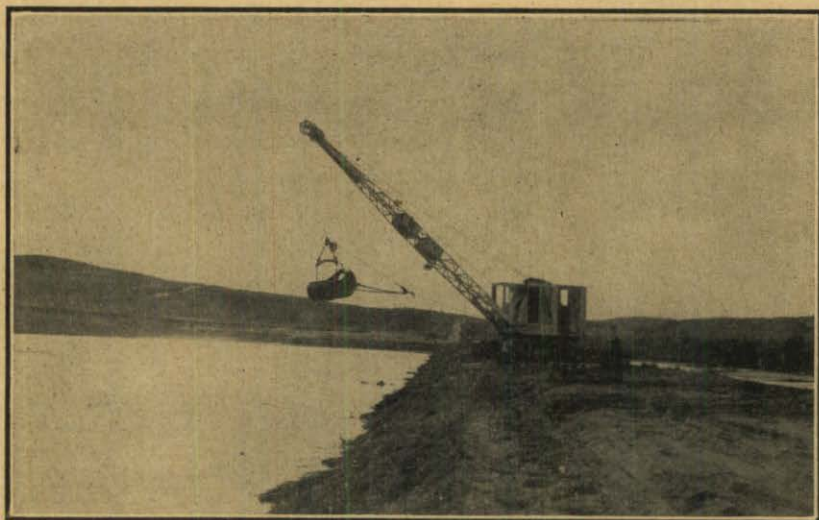
Drag-line work thru lake in Lakeside-Ellsworth project. This is the kind of material also used to cover the sand base as shown in the picture below.
