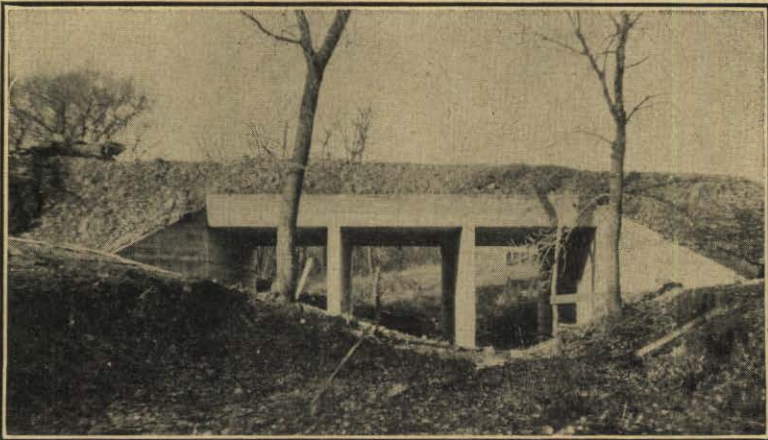
Three steps in replacement of timber bridge. Project No. 97-C.
