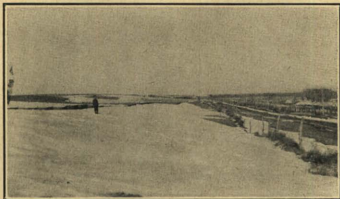
Above is a view of the State Highway in right hand side of picture, protected by snow fence, which is shown on left hand side of picture.
