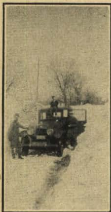
View below is a road which had not been protected by snow fence. Note car in the drift.
