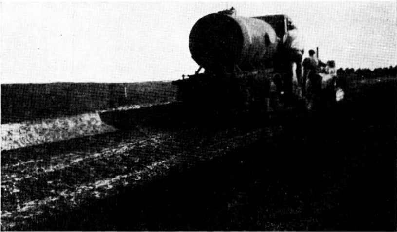
A pressure distributor used for application of oil.
