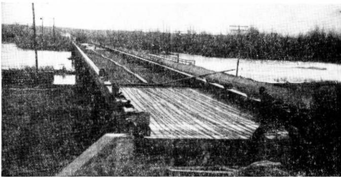
Views of a typical transverse joist girder bridge, over the South Platte river, near Ogallala.
