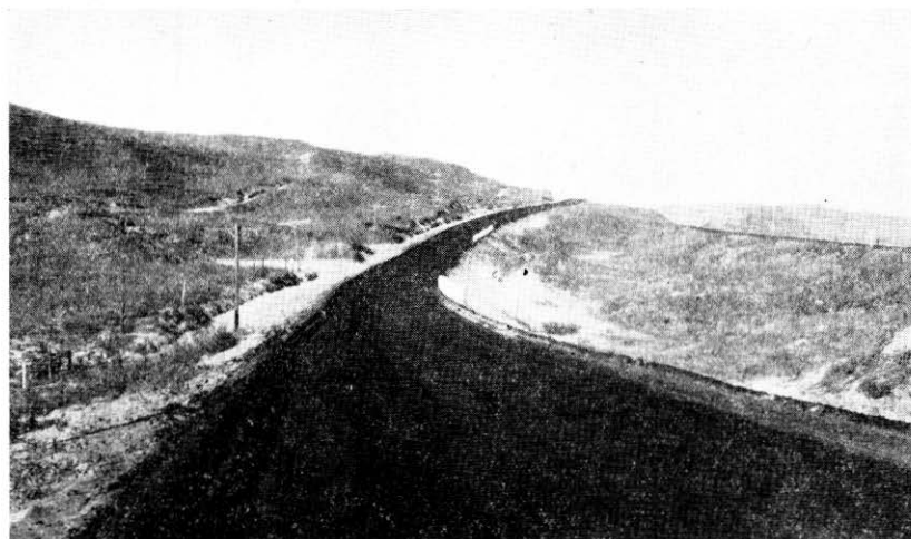
Oiled gravel road near Whitman, Grant County, on the Potash Highway.
