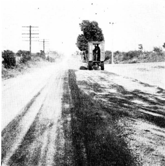
Soaking up oil with light application of gravel.
