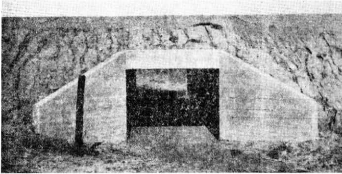
Single Box culvert Harlan County.
