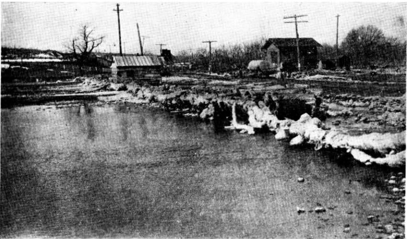
High water on Highway No. 75, near Union.
