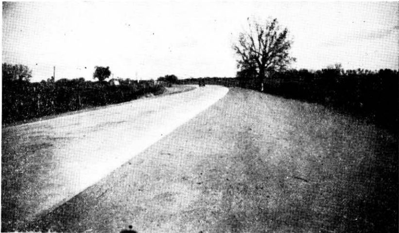
Long, superelevated curves are built on paved roads for the convenience and safety of traffic. This view is south of Saint Paul.
