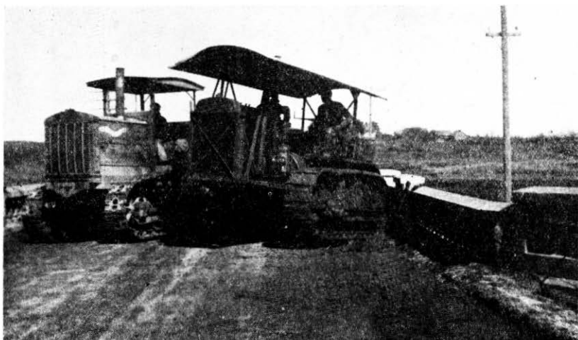
Testing strength of old concrete slab bridge, south of Nebraska City. Project 2-C.
