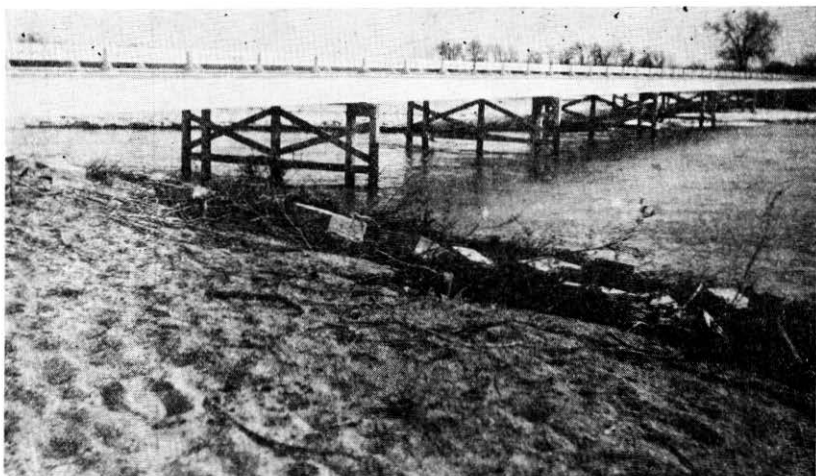
Alda state aid bridge over south channel of the Platte river. Project 860.
