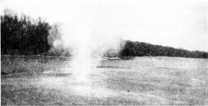
Ice fields on the Platte river are broken up by dynamite for the protection of the bridge piers.
