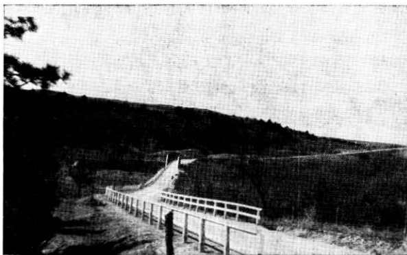
Wood guard rail. This type is being replaced by woven wire, and cable guard rail.
