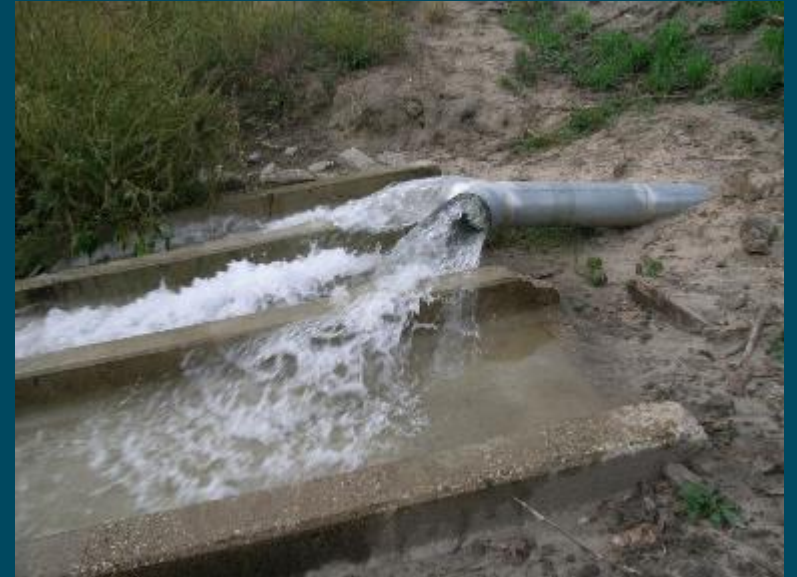
North Dry Creek Streamflow Augmentation Project, TBNRD
