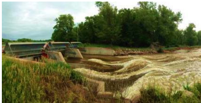
30-Mile Canal Headworks, June 2015
