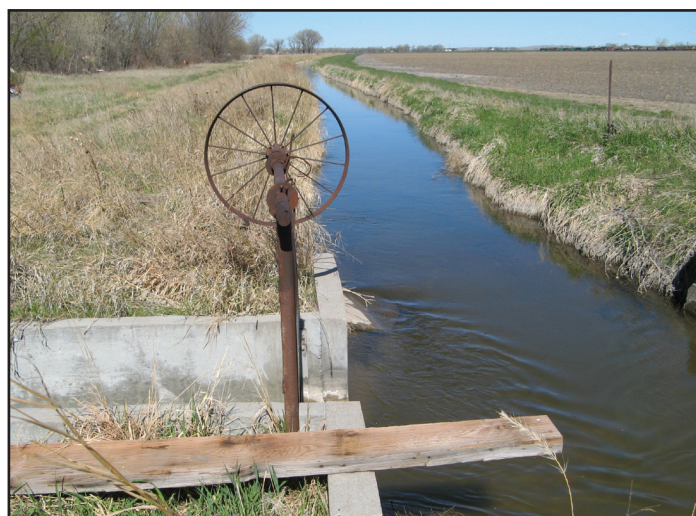
Image 3: Photograph of a filled canal during the groundwater recharge demonstration project.
