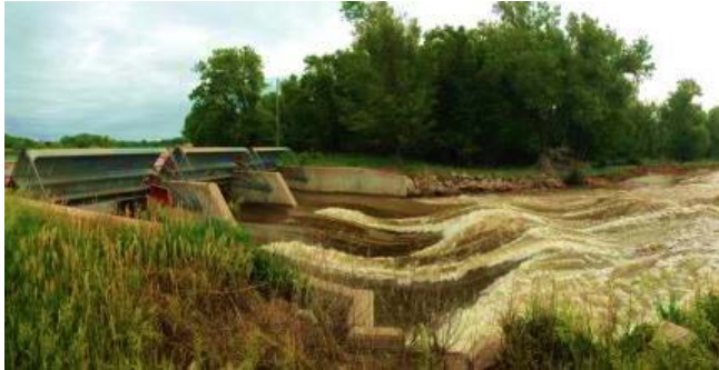
30-Mile Canal Headworks, June 2015
