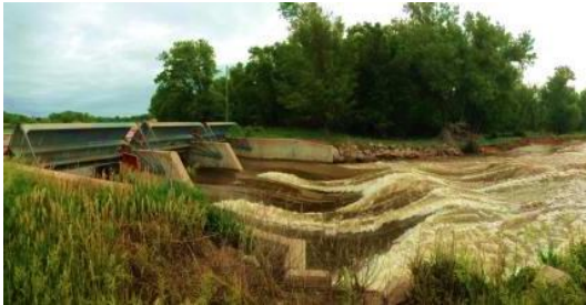
30-Mile Canal Headworks, June 2015
