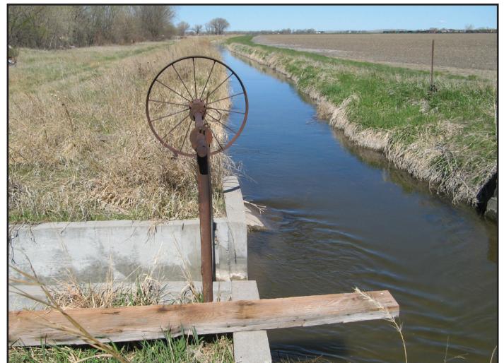
Image 3: Photograph of a filled canal during the groundwater recharge demonstration project.
